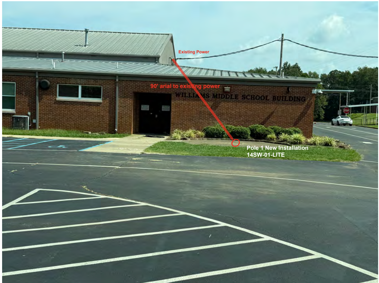
Light pole 1, location
